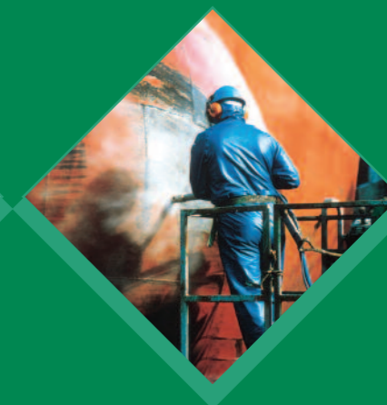
UHP Water Blasting
